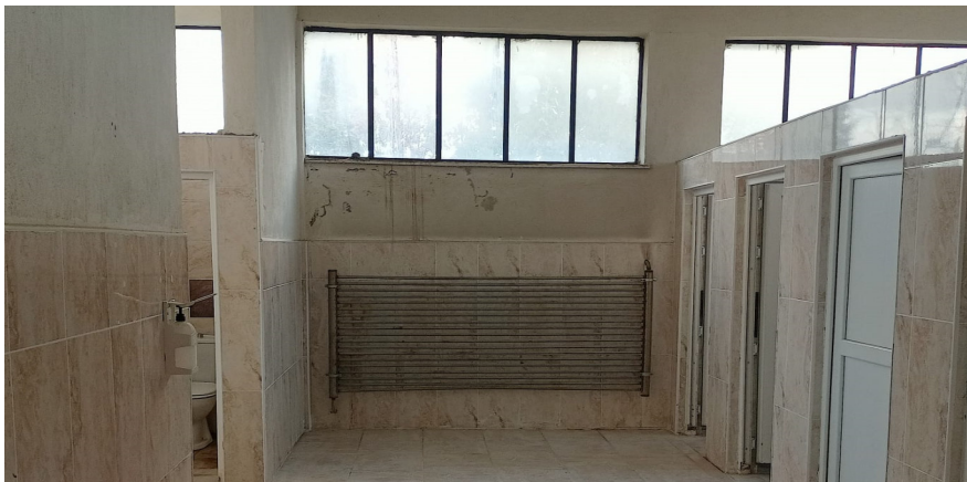
Figure 3: 3rd Stage Studies for Space Heating with Deaerator Exit Steam from Waste Steam in Ammonia Nitrate Production
