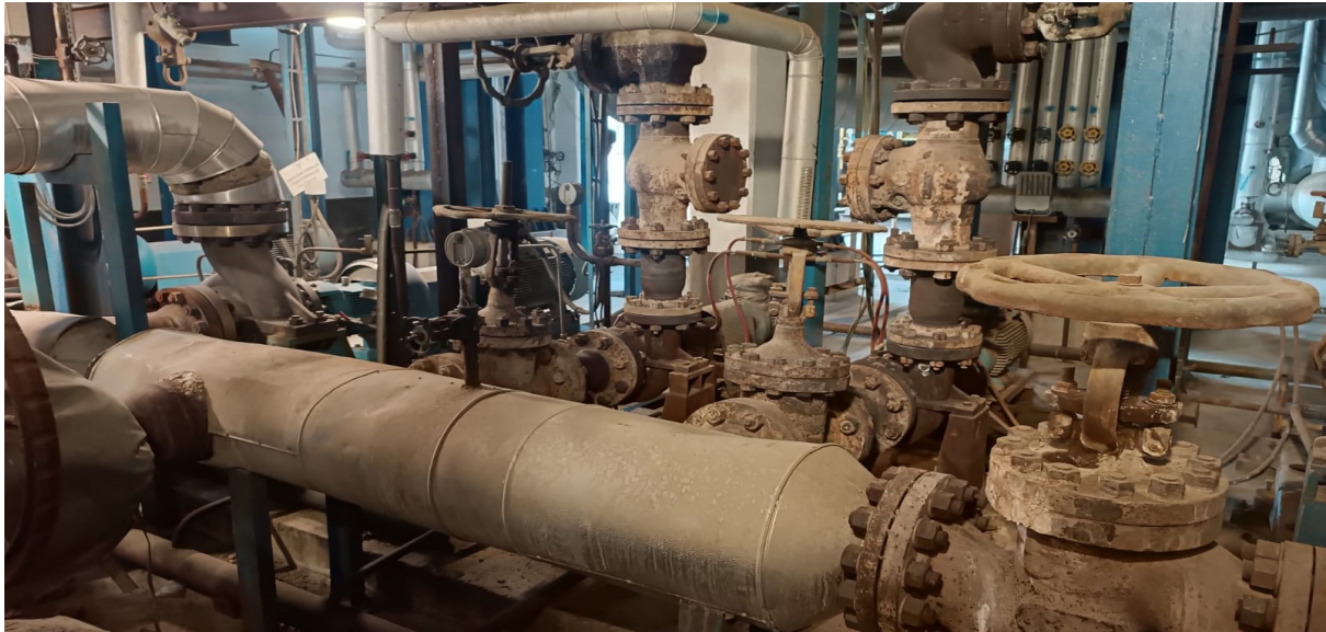
Figure 3. Circulation Pumps Before Revision (180 t/h)
